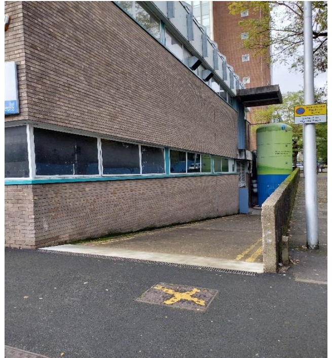
Down the ramp leading to the prayer room entrance
